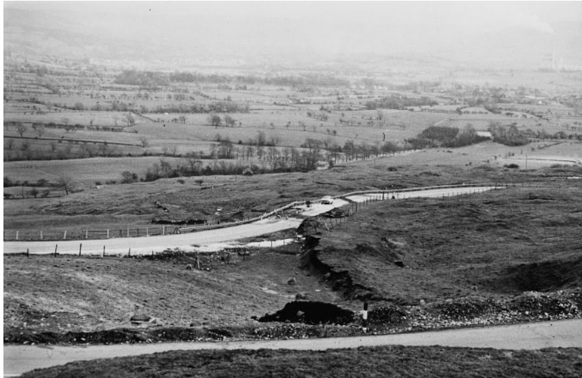
Fig. 6. The northern margin of the landslide where the slide debris is heaved obliquely up the rising slip surface to create a fresh and rising step in the ground surface. The photograph was taken looking down the slide in early 1977, when the movement rate was at a maximum; the scar is now less active and is largely grassed over.
