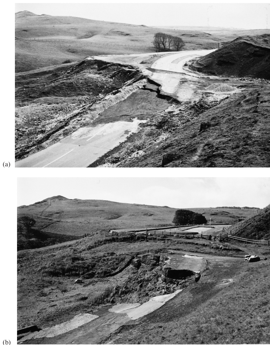
Fig. 5. The breaks in the upper road surface where it crosses onto the active landslide from the southwest. Photographs were taken in (a) 1977, soon after the road was closed to traffic, and (b) 1998. The earth bank across the road below the fence was placed over the landslide's marginal scar in 1990, and has subsequently broken.
