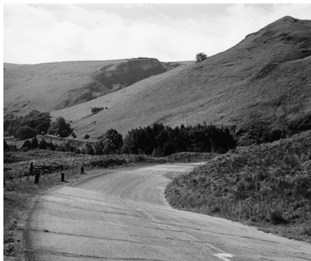
Fig. 10. Severe distortion without major fracturing of the lower road across the debris flow elements of the landslide in 1998.
