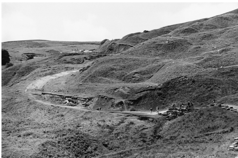
Fig. 9. The upper road across the landslide is broken by the head scars of element M as this cuts into the stepped and hummocked ground created by the multiple slide blocks which form element H, as seen in 1998.
