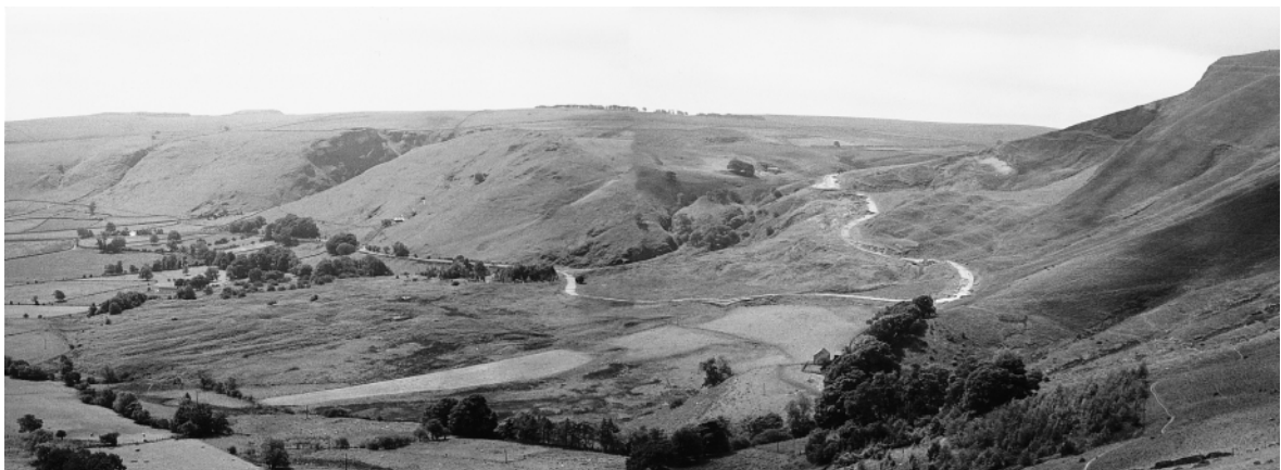
Fig. 2. The Mam Tor landslide viewed from the sandstone ridge to its north in 1998. The head scar is only seen in profile on the right, with the Iron Age fort ramparts visible just below the skyline. The road descends over the slipped blocks of the landslide mass, before turning back across the lower debris flow. Treak Cliff is the steep slope in reef limestone extending from the far side of the landslide to the shadowed breach of the Winnats Pass.
