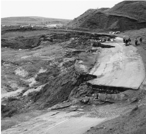
Fig. 16. Severe damage to the upper road on the southern part of the landslide, as it was in 1998. The road has slide element L falling away to its left, and steps down onto element J in the foreground. Intermittent remedial works have set the road further into the slope, creating the steep bank with trench drains on the right; the same works have placed fill to support the left of the road, but have therefore head loaded the active landslide element L.
